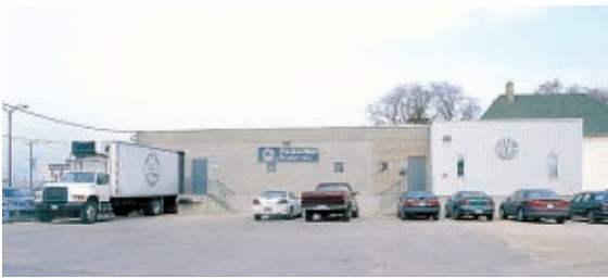
To-Le-Do Foodservice Production Plant, 143 Henry Avenue, Winnipeg.
